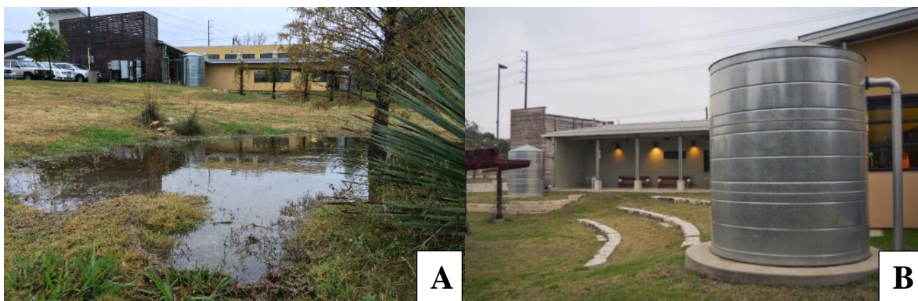
Figure 1 – Twin Oaks Library (A) Rain Garden and (B) Cisterns
