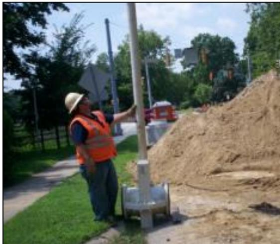
Figure 4. Installation of a valve for an auxiliary throttle valve
